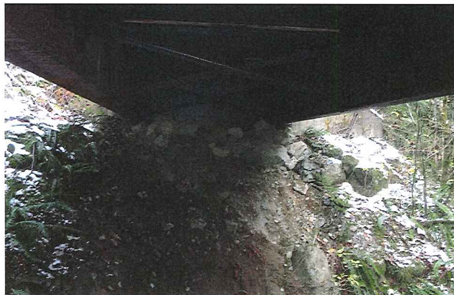
CK-2025 Abutment Left Bank
