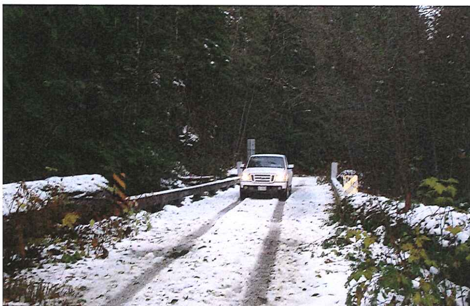
CK-2025 Approach Right Bank
