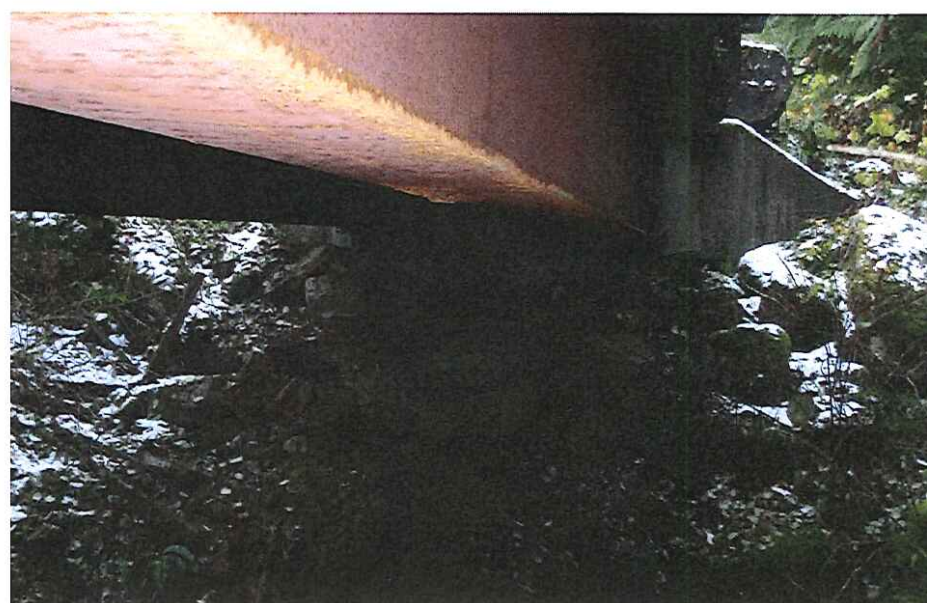
CK-2025 Abutment Right Bank
