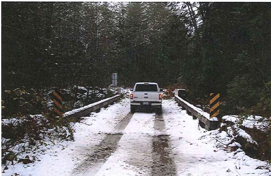
CK-2025 Approach Left Bank
